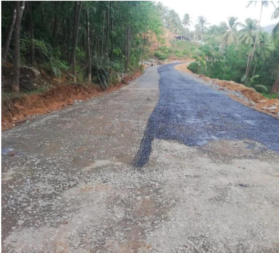
Plate S-6: Quarrying Road
